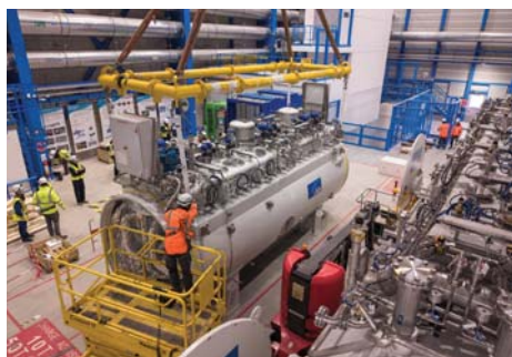
The new cold box transported to the underground tunnel of the HLumi LHC, near the ATLAS experiment. Credit: CERN
