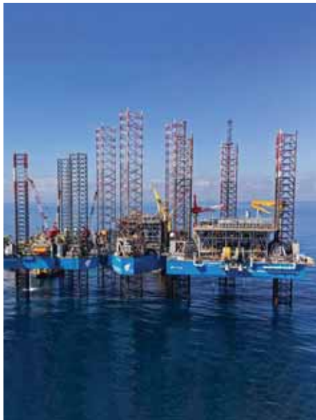
Chart's Integrated Pre-Cooled Single Mixed Refrigerant (IPSMR®) technology enabled the first LNG production at New Fortress Energy's Fast LNG project in Altamira, Mexico. Credit: New Fortress Energy
