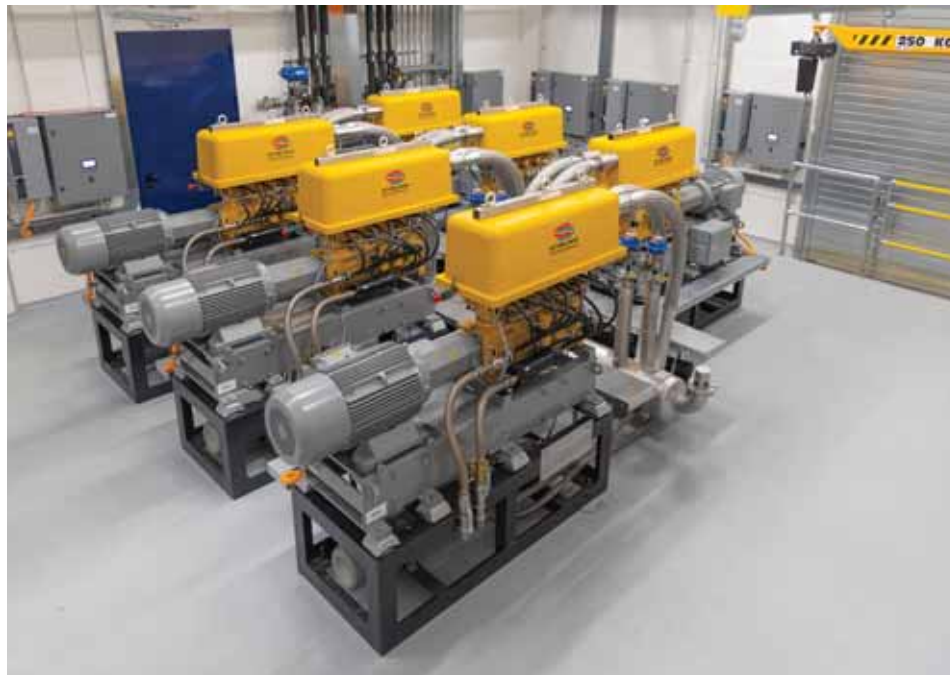
2019 Stirling Cryogenics hydrogen reliquefier for cold neutron source at RID. Credit: Stirling Cryogenics
