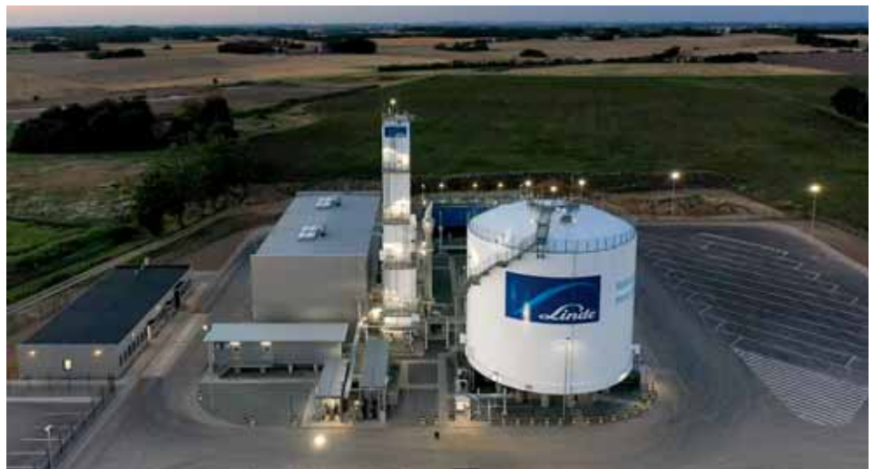
Linde's FLEXASU plant in Denmark, designed to operate and store products when wind energy is abundant and less costly, meets the entire demand for Denmark. Credit: Linde
