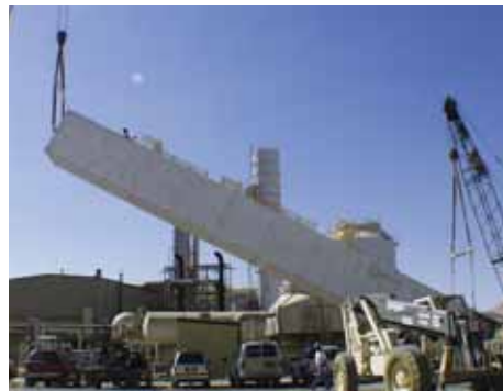
Removing an ASU cold box. Credit: Nils Tellier
