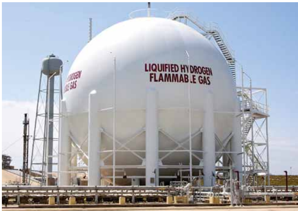
Liquid hydrogen storage sphere at KSC. Credit: GenH2
