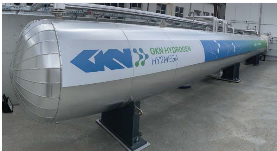
GKN's HY2MEGA is the largest metal hydride storage unit on the market and ideally suited for energy supply applications where safety and compactness are crucial. Image: GKN Hydrogen
