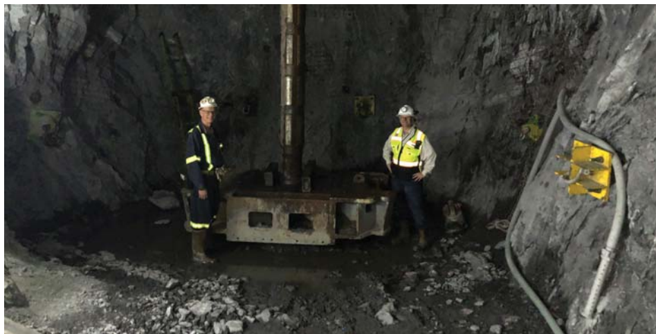
Drilling the ventilation shaft. Fermilab's Syd Devries (left) and James Rickard stand with the reamer. Image: Andrew Hardy, Thyssen Mining
