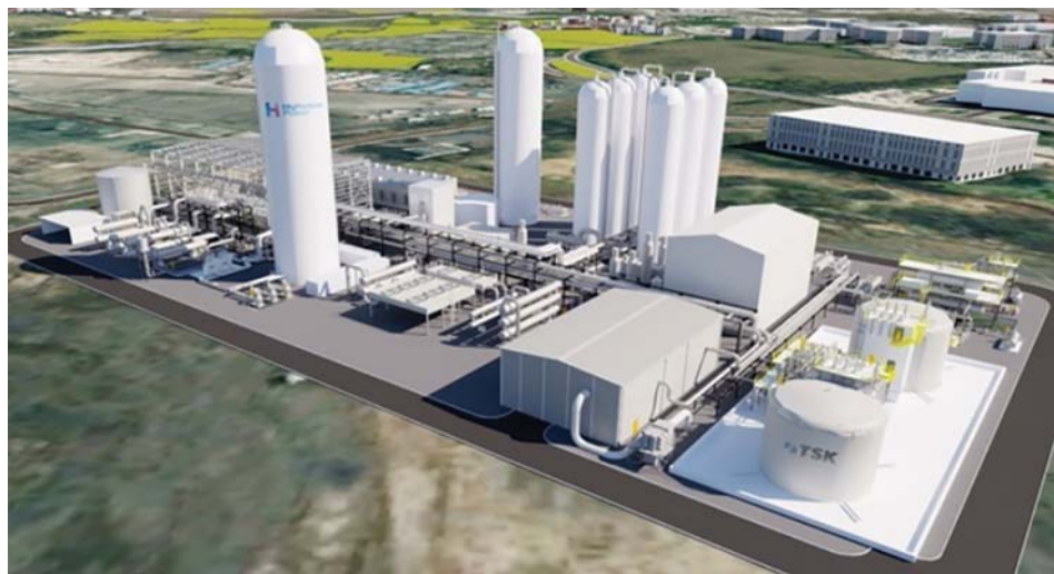
Rendering of a 50MW / 300MWh liquid air energy storage plant in Manchester, UK. Credit: Highview
