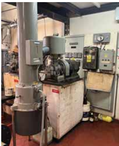
Stirling Cryogenics liquid nitrogen system at Universidad de Buenos Aires - Argentine dated 1958. Credit: Stirling
