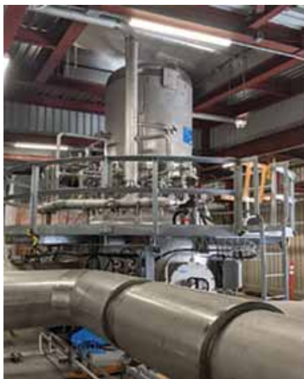
Transfer lines and distribution boxes Credit: SLAC
